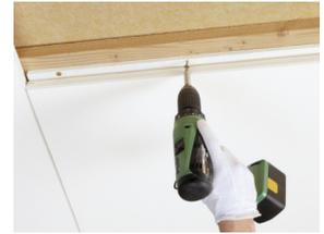
Master F is installed by screw fixing
