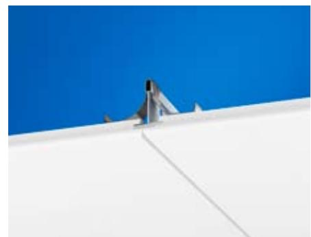
Hygiene Labotec Ds C1 section with Connect Hold down clip Ds
